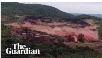
Dam Collapse, Brazil, 2015-2019
