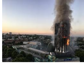
Grenfell tower in London, UK, in 2017
